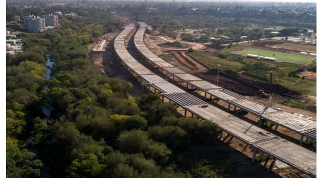
Road - Córdoba City Beltway (City of Córdoba)
